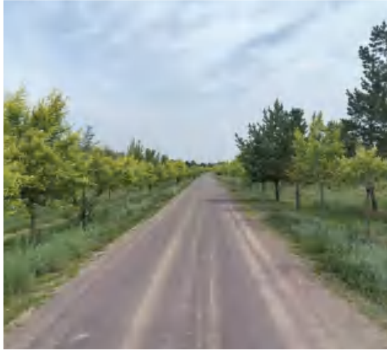
Figure 3. A mixed protective forest of Scots Pine and Golden Elm planted along both sides of the 4-km sand-crossing road, serving both road protection and landscape enhancement purposes
