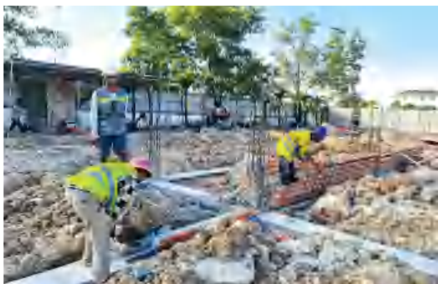
Construction work of the project in Cambodia Photo by IRD
