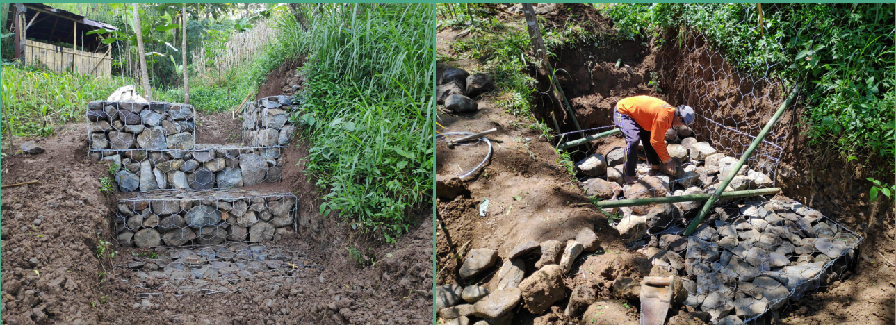
Gully-erosion control structures used in the project – gabion (left) and bamboo and gabion (right). Photos: Watershed Management Technology Center
